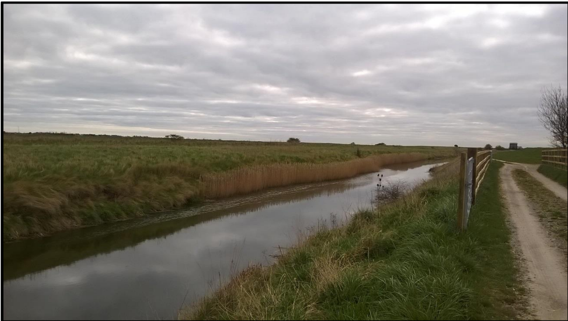
Plate 8.2b: Winestead Drain, looking downstream towards WOPS.
