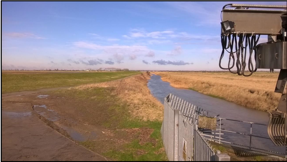
Plate 8.2a: Winestead Drain, looking upstream from WOPS.
